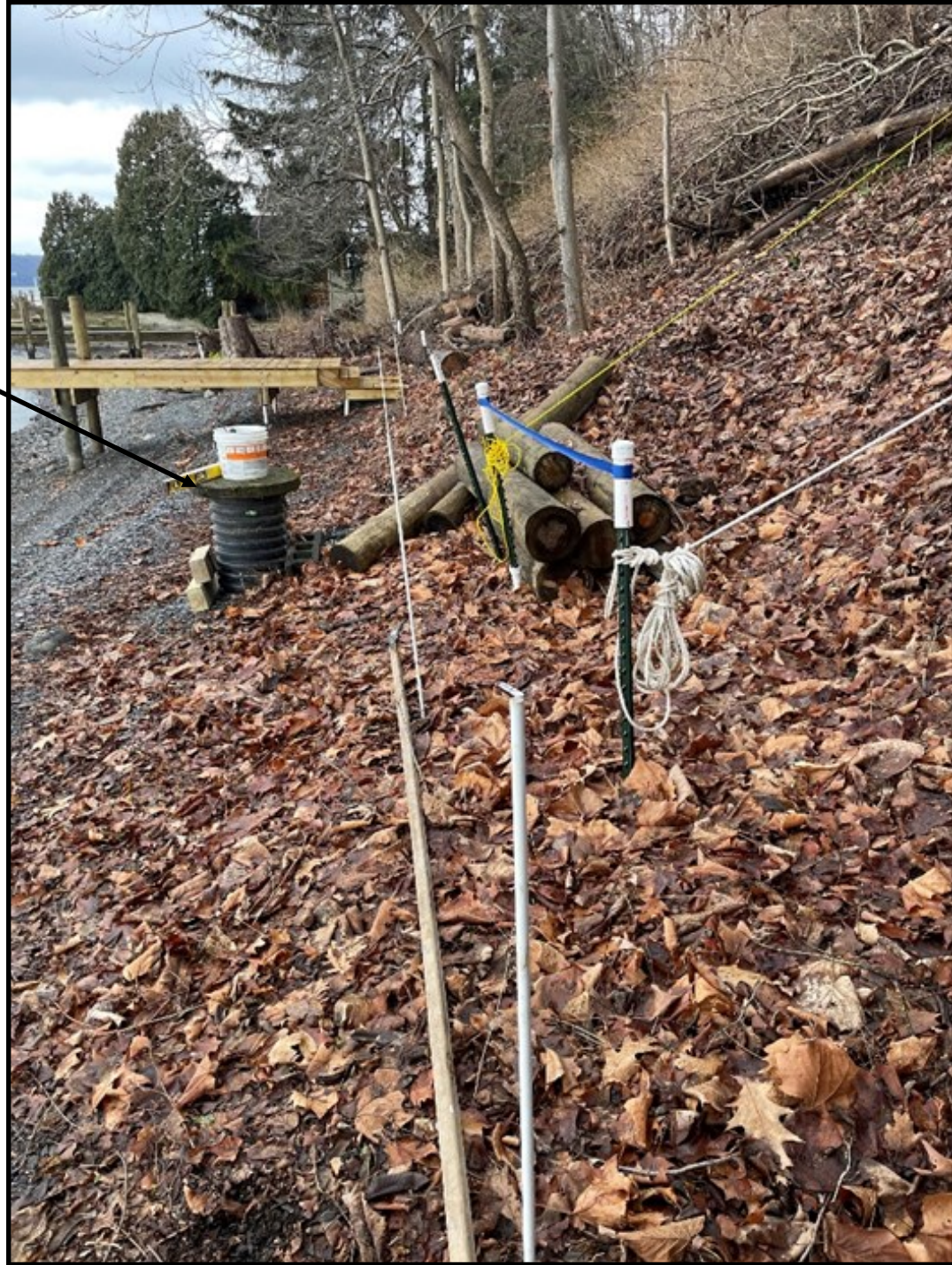
The white stakes mark the edge of the 100 year flood plain (386.0') —Tram will terminate at the green markers above the plain
