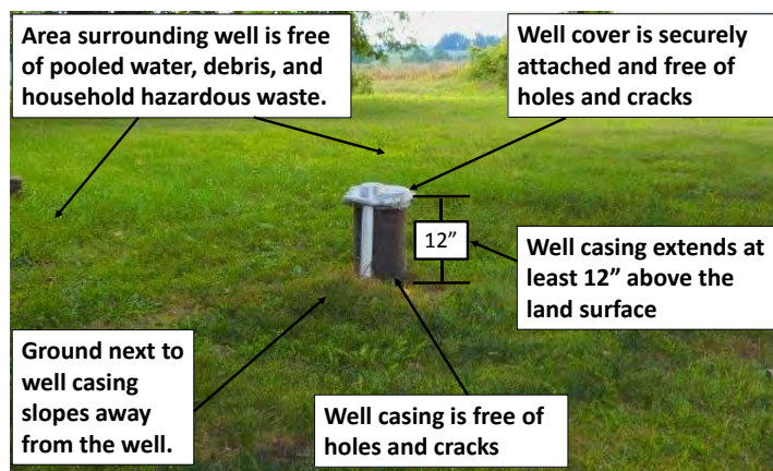
Figure 1: Photo of a properly constructed well.
