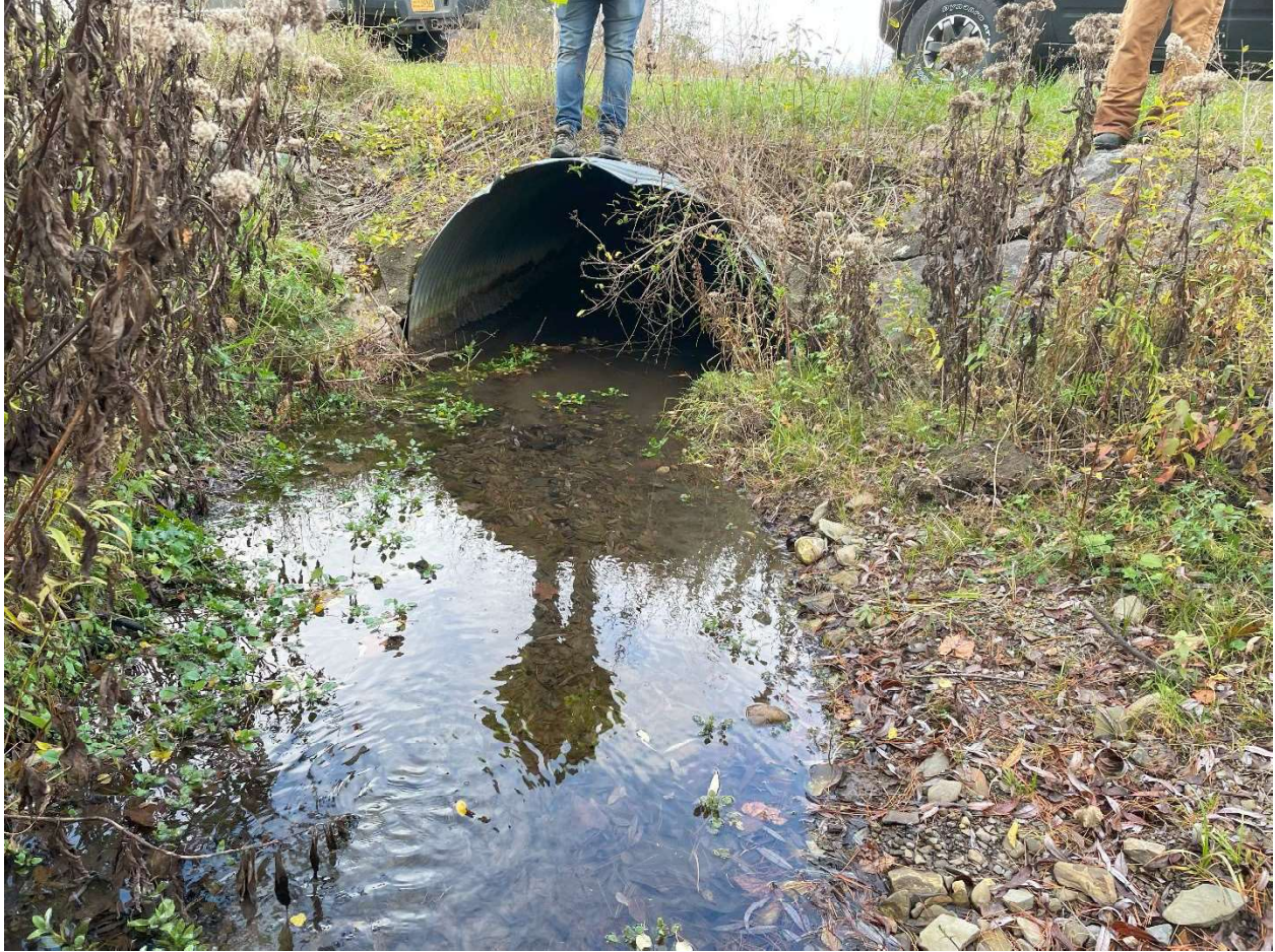
Figure 11. Agard Road culvert looking north.
