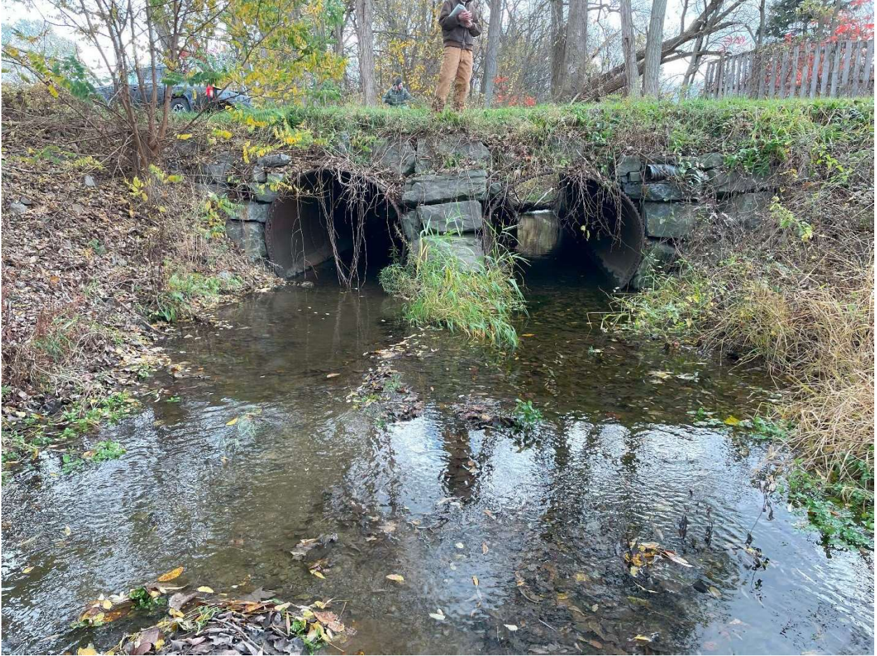
Figure 17. Reynolds Road culverts looking north.
