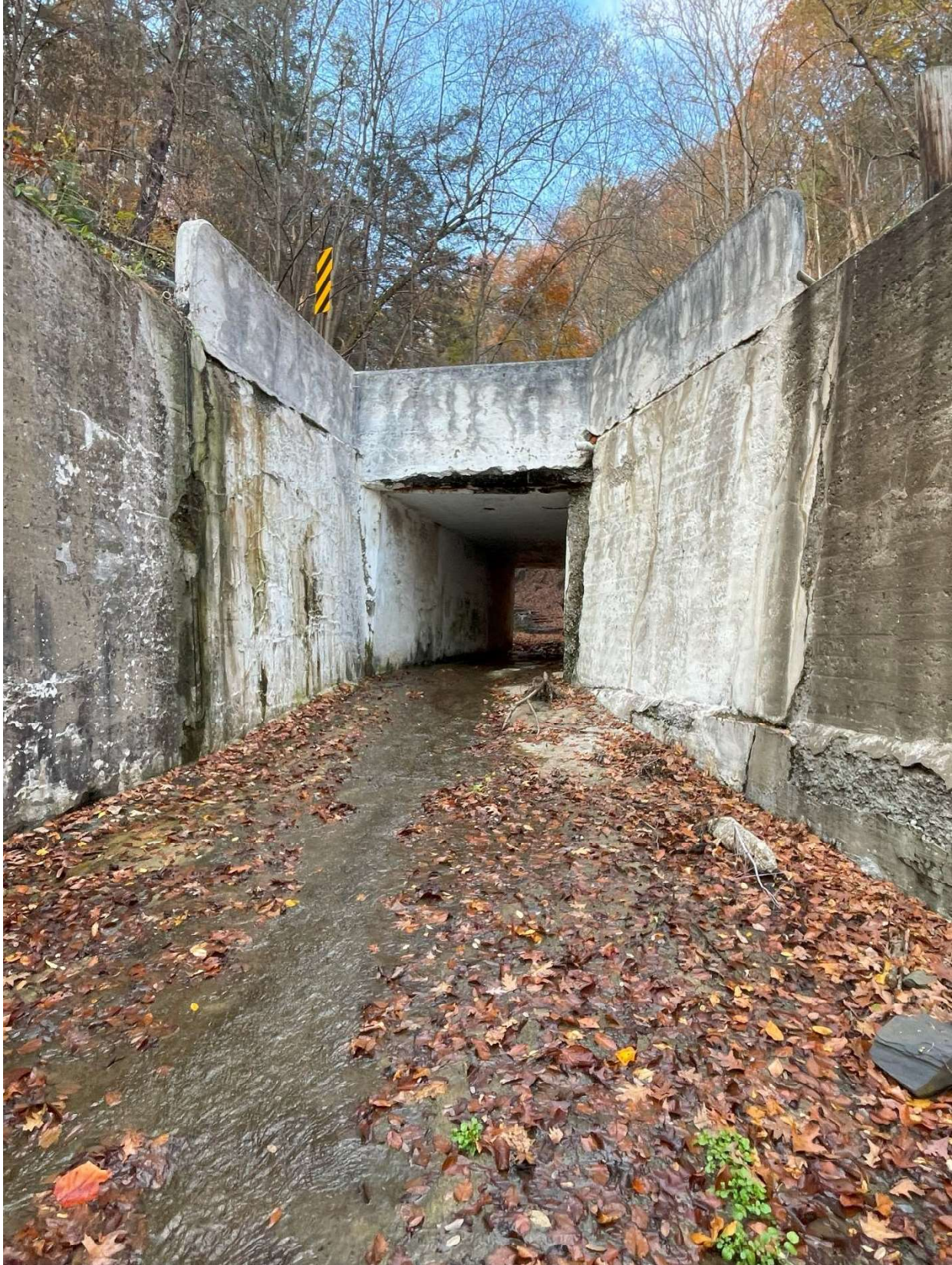
Figure 4. Maplewood Road culvert looking west.
