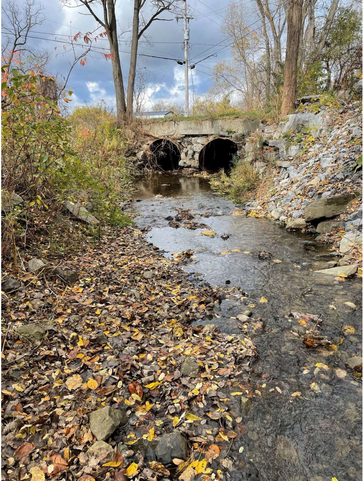
Figure 18. Reynolds Road culverts looking north.
