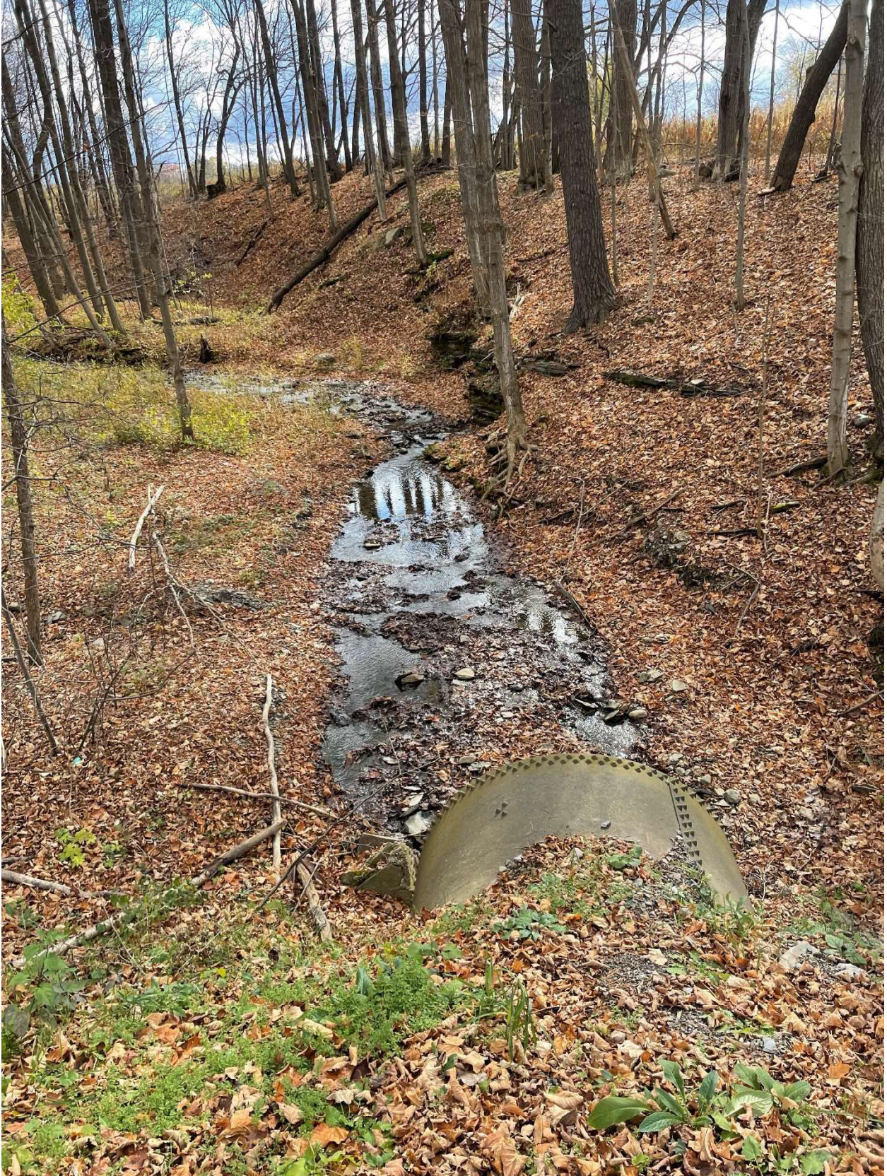
Figure 22. Iradell Road culvert looking south.
