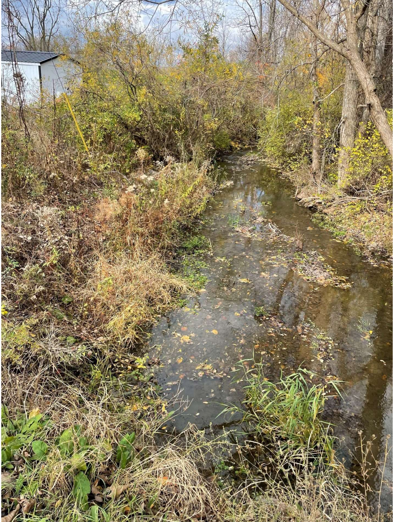
Figure 19. Reynolds Road culverts looking north.
