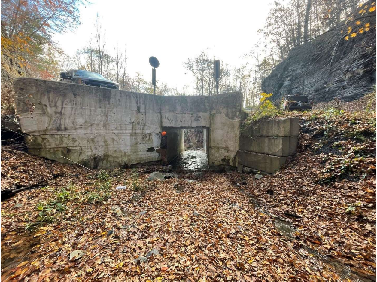
Figure 2. Maplewood Road culvert looking east.
