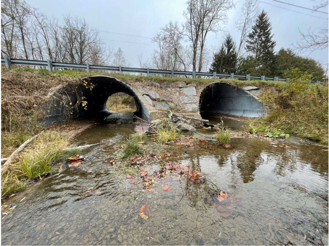
Figure 16. Curry Road culverts looking north.
