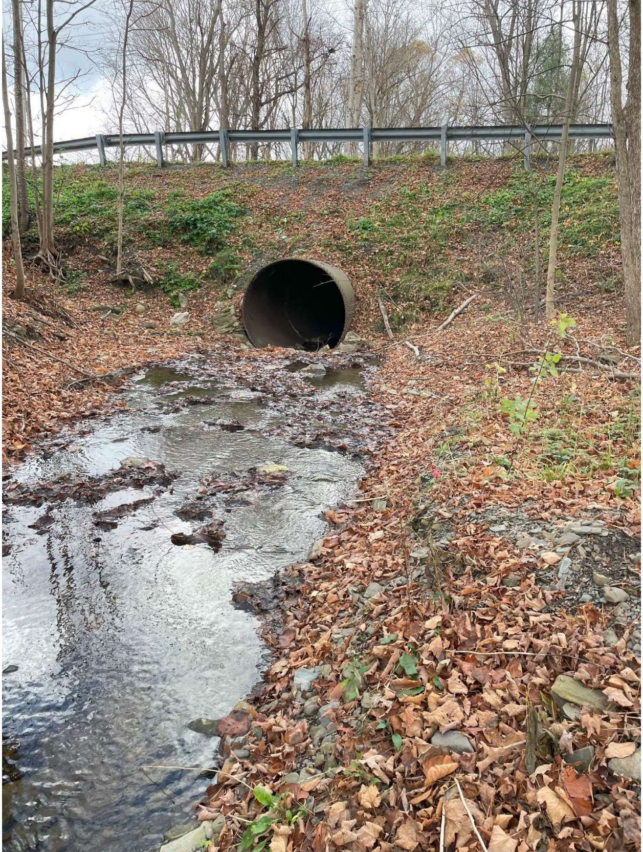
Figure 23. Iradell Road culvert looking north.
