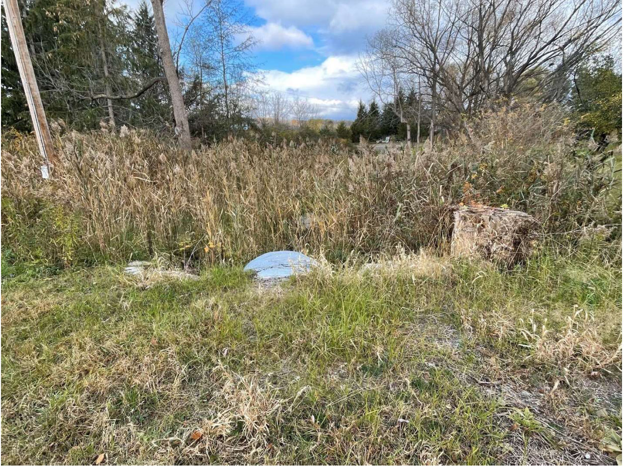
Figure 12. Agard Road culvert looking north.
