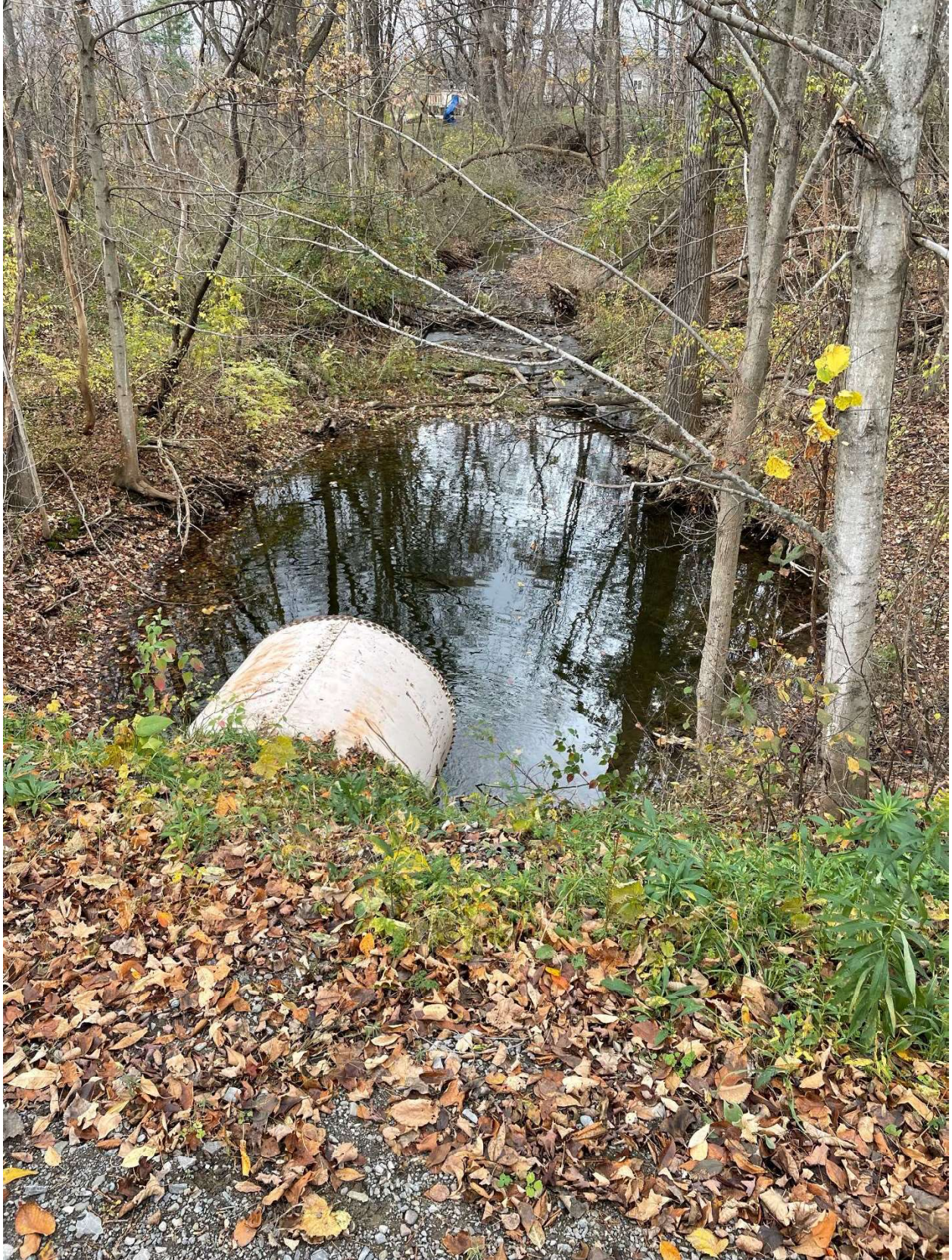
Figure 29. Iradell Road culvert looking north.
