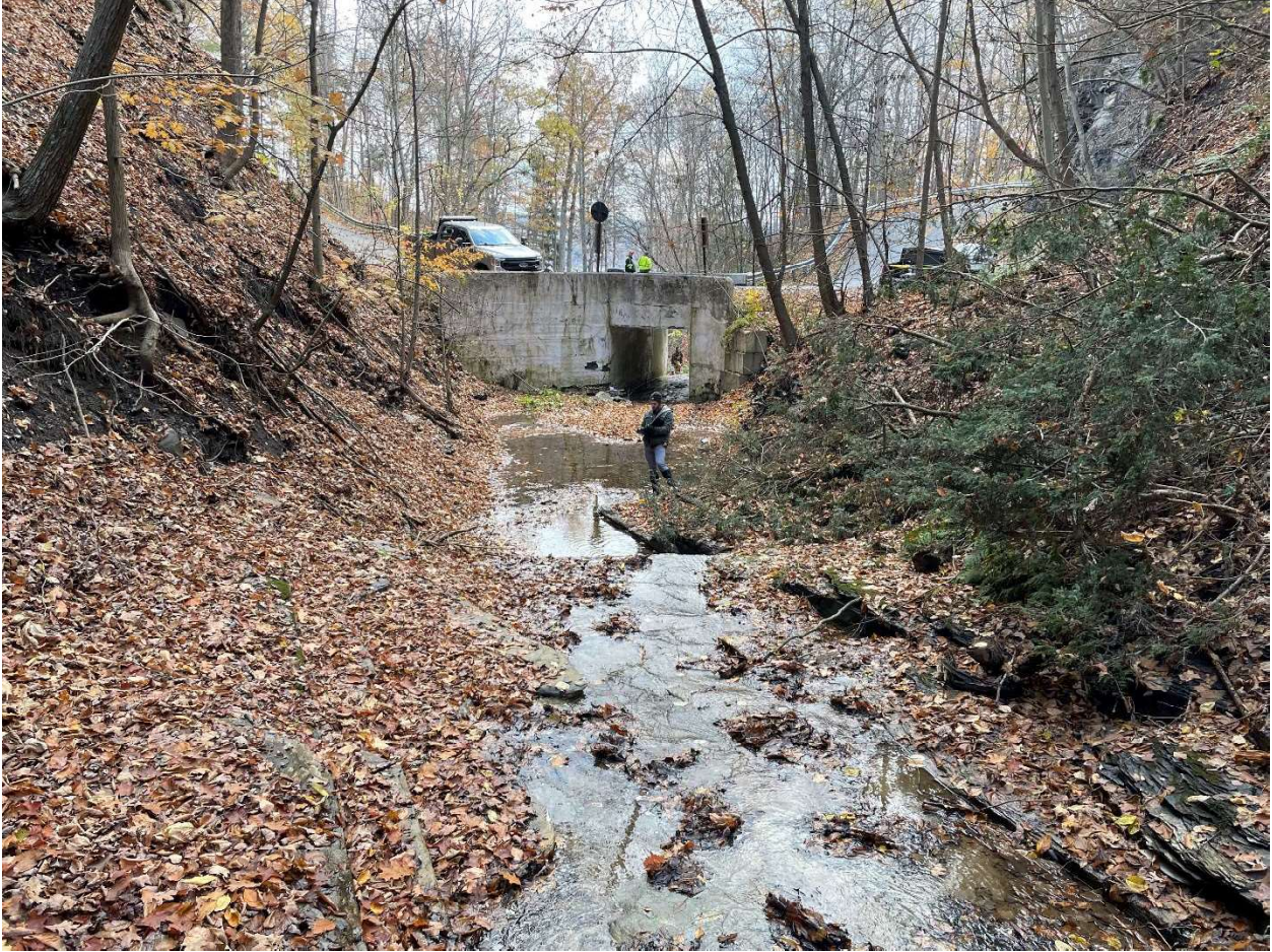
Figure 5. Maplewood Road culvert looking east.
