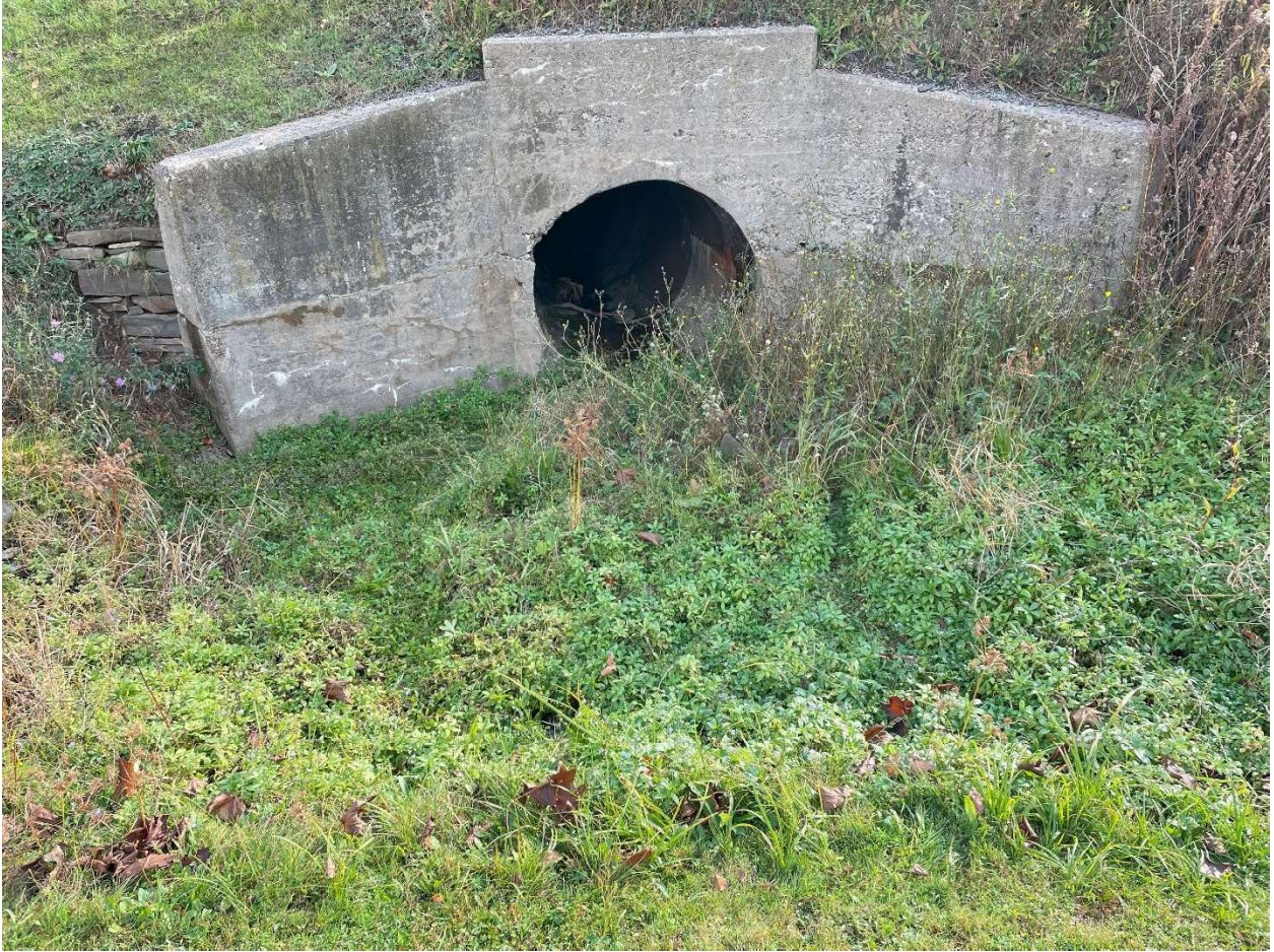
Figure 10. Garrett Road culvert looking east.
